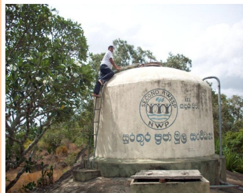
Fig.2: A typical "Seed" (Solar panels, DC water pump and storage tank) necessary to start and grow a solar village, providing the initial income source.
