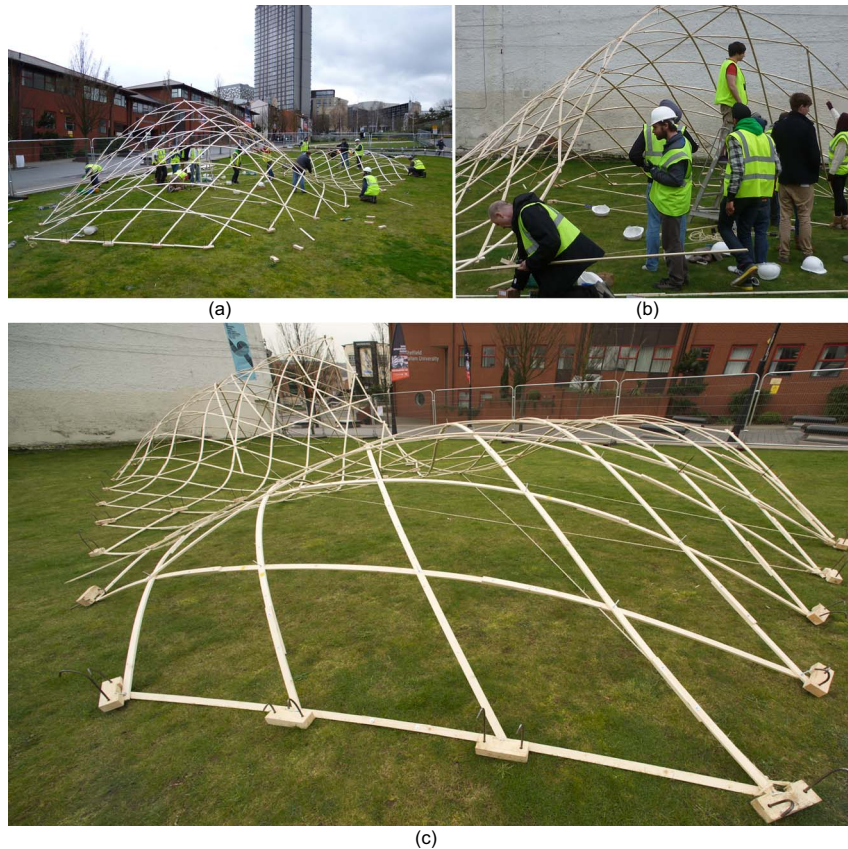
Figure 10. (a): The geometry of the structure was stabilised by bracing and triangulation. (b): The swells nearing completion. (c) The swells on display at Sheffield City Centre
