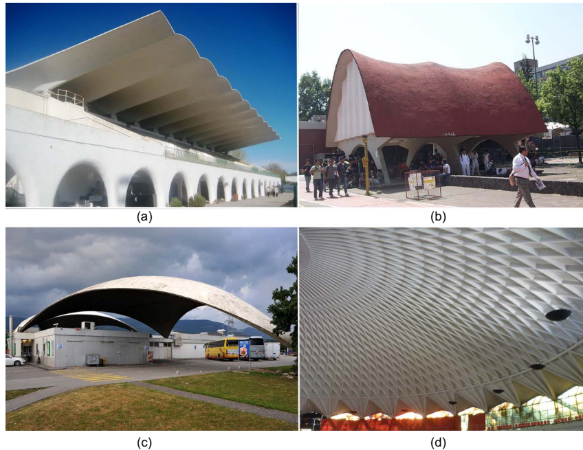
Figure 4. (a) Thin repeated concrete shells form the canopy of La Zarzuela Hippodrome roof by Torroja [By Outisnn (Own work) (GFDL ( http://www.gnu.org/copyleft/fdl.html ))), via Wikimedia Commons]. (b) Cosmic Ray Pavilion, Mexico City by Felix Candela (1951) [By GAED (Own work) [Public domain], via Wikimedia
