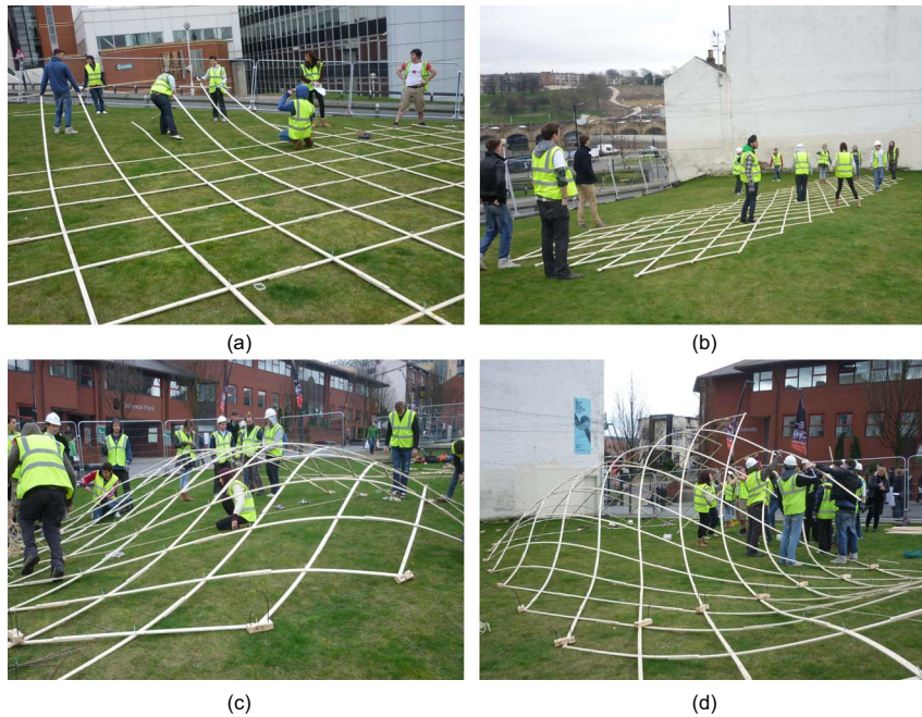
Figure 9. (a) The gridmat was constructed flat on the ground by splicing timber laths. (b) The gridmat was stretched and shifted into position. (c) The gridmat was compressed to form the baby swell. (d): The mother swell is formed
