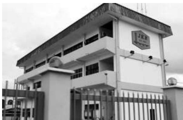
Figure 1.5: Example of standard JKR building (1957). Source: Author
