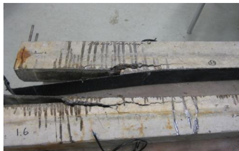
Fig. 10 Debonding of CFRP fabrics after load testing
