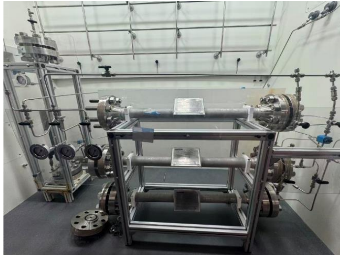
Figure 3. Hydrogen pressure tube system.
