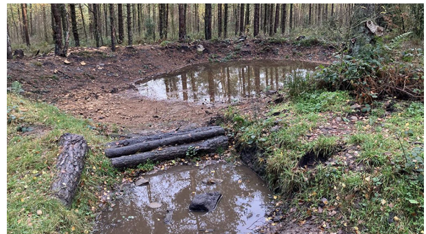
Fig. 3 Lady Cannings Plantation attenuation pond with sediment trap
