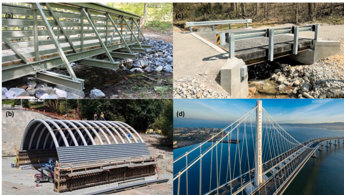
Fig. 11. Different structures designed using composite materials, showing (a) Composite lightweight pedestrian bridge. (Image credit: Bedford Reinforced Plastics. Source: [210]), (b) Glass Fiber Pultrusion Bridge, Washington, USA, (c) Composite lightweight bridge in Morgan County (Image credit: IACMI. Source: [211]), and (d) The East Span of the San Francisco-Oakland Bay Bridge, USA (Image credit: TyLin).
