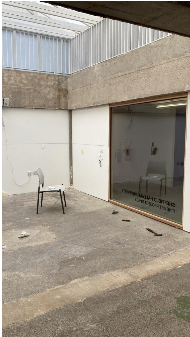
Figure 86. S1 Space work in progress with material placements, S1 Art Space Day 1 (2022)
