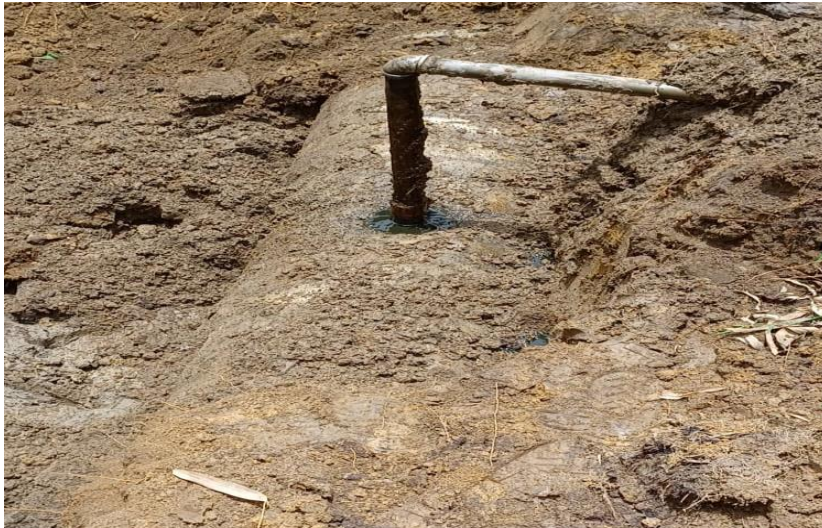
Figure 1. 7: Suspected illegal oil siphoning activities from a pipe transporting crude oil
