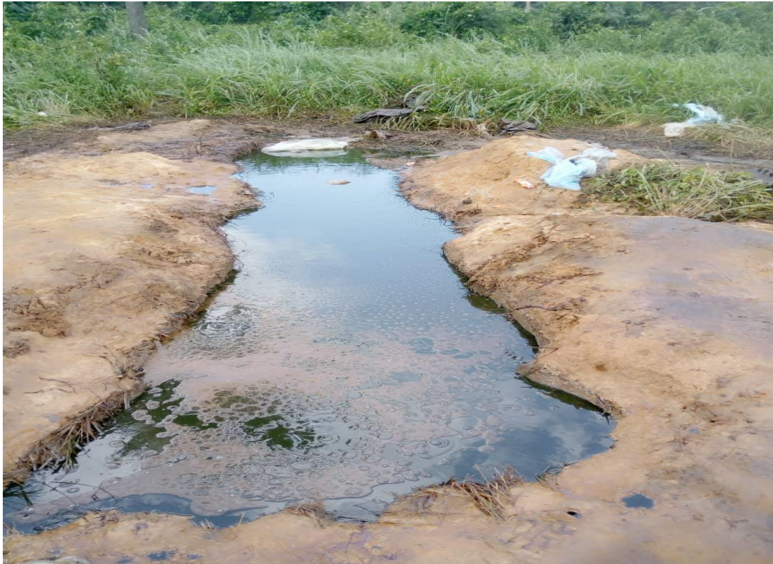
Figure 1. 5: Leakage from a suspected sabotaged underground pipeline
