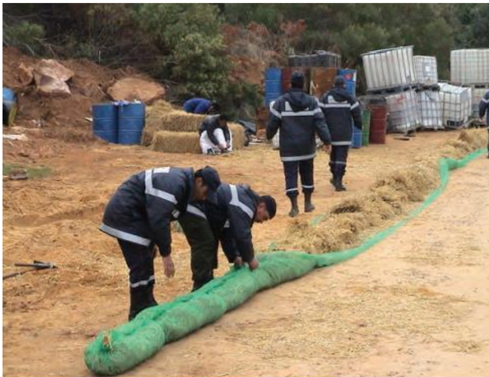
Figure 2. 2: Improved adsorbent boom constructed from netting and straw Source: (59)
