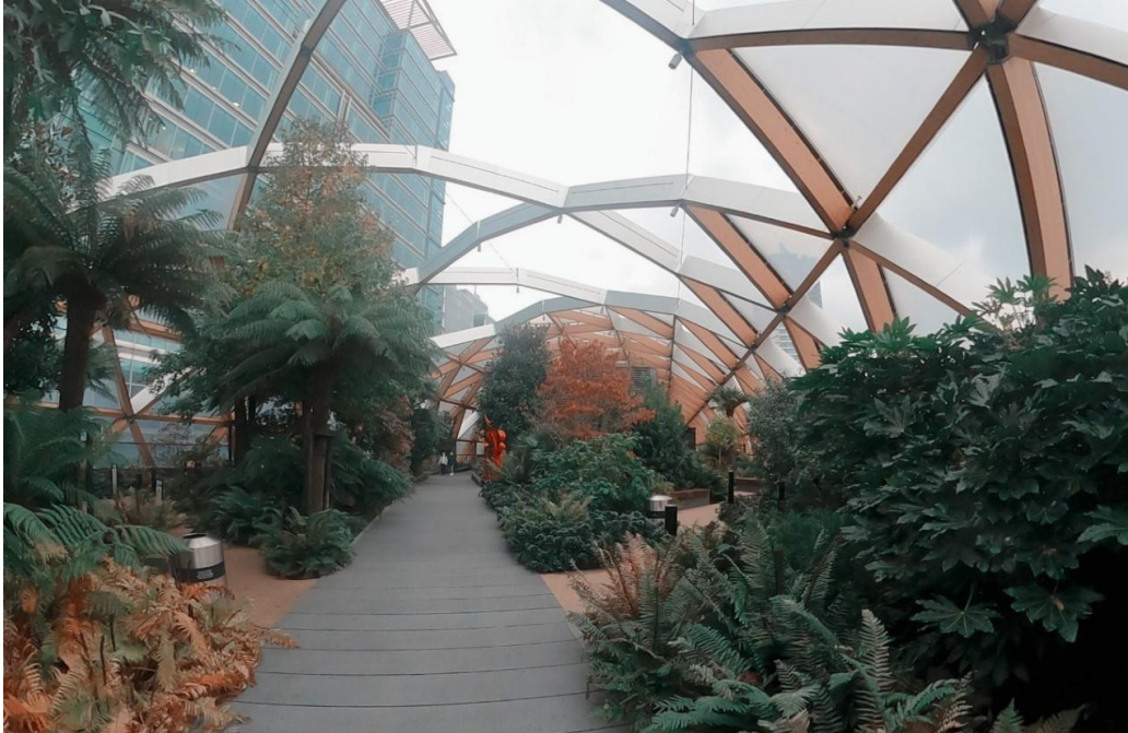
Fig.2. Crossrail Place roof garden, Canary Wharf, London. Source: Author.
