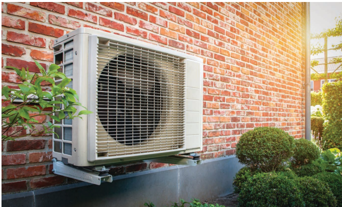
Image shows a wall mounted ASHP. Source: Our Heat Pump Packages | Lochinvar
