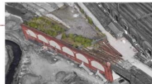
TOP VIEW OF THE ARCHES
