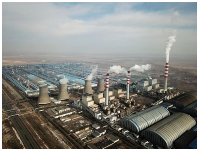
Figure 11. Xinfa Group Xinjiang Branch Company facility in Wujiaqu, XUAR. Source: Shandong Provincial People's Government Office in XUAR, Online .
