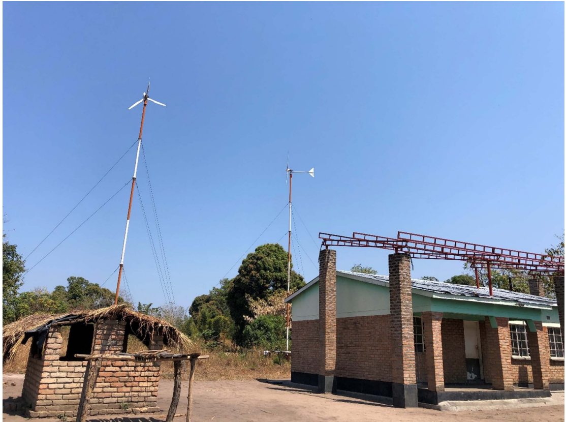
Figure 7. Abandoned solar PV-wind mini grid infrastructure at Mdyaka ( source: authors' own ).
