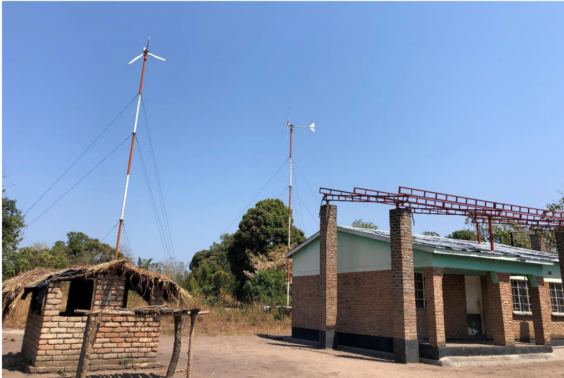
Figure 7 Abandoned Solar PV-Wind mini grid infrastructure at Mdyaka (Source: Author's own)
