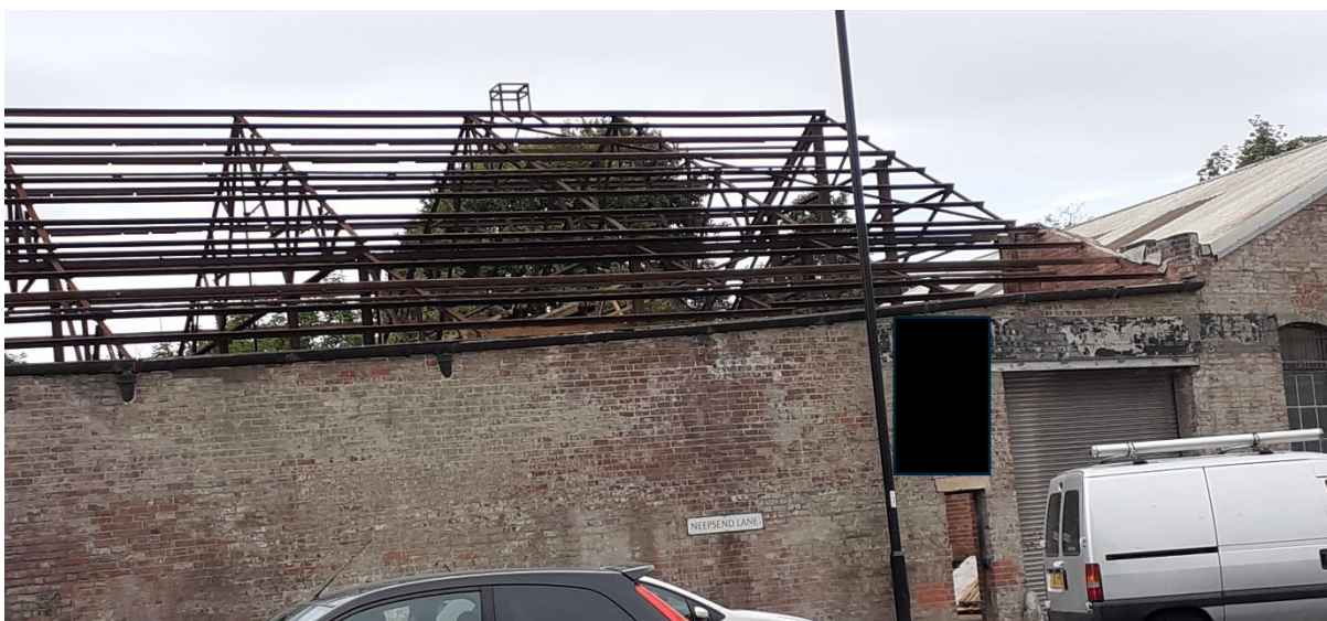
Figure 6.7 Before Picture: Radiac Works as a derelict shell. 23 07 2020. Charlene Cross.
