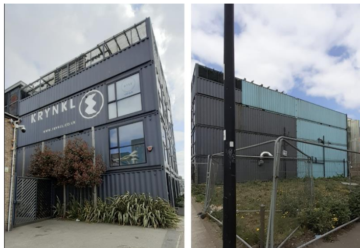
Figure 4.7 Meanwhile Uses: a building composed of shipping containers. Both images were taken on 25 04 2021. Charlene Cross.
