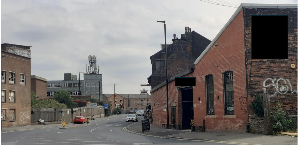
Figure 6.8 After Picture: Radiac Works restored and made habitable (right). The Cannon Brewery (left) is across the road. Neepsend Lane. Charlene Cross. 25 07 2021.
