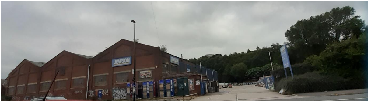
Figure 5.16 Actively occupied building. Corresponds to HELAA site S03239, Mowbray Street. Trees to the right separate this site from the former concrete works- HELAA site S03238- next door. 25/08/2021. Charlene Cross.
