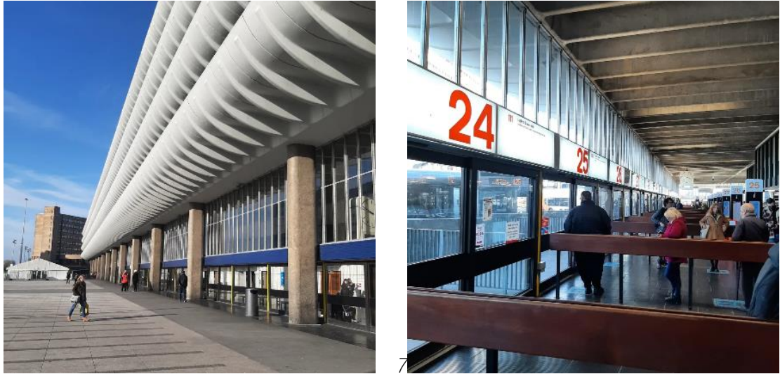
Figure 2.2 Preston Bus Station, 17 th March 2022.
