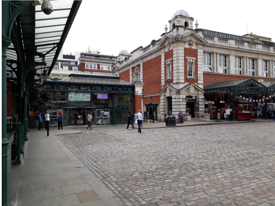
Figure 4.3: Entry to the LTM off Covent Garden.
