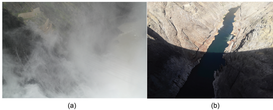
Figure 8. Power house and transmission cables of Tekeze hydropower a) during spilling and b) normal operation.
