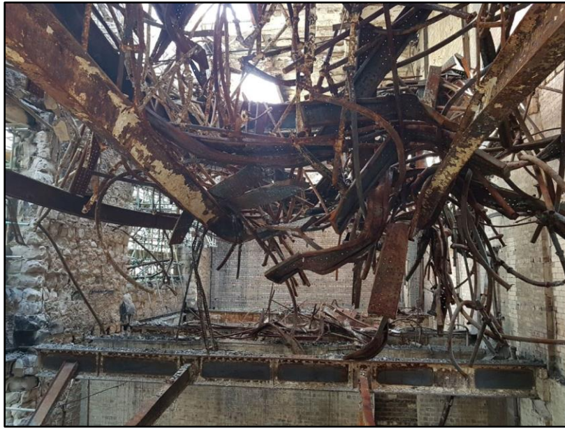
The interior of the Mackintosh Building after the 2018 fire (photo 2019).
