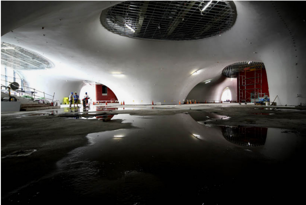
Figure 1: The unusual cavernous spaces of Taichung Metropolitan Opera House [www.DesignBoom.com]
