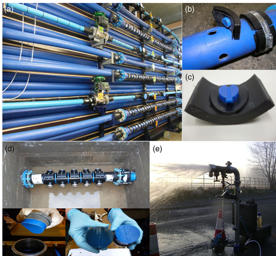
FIGURE 1 (a) Real-scale DWDS laboratory facility at Sheffield University, (b) PWG coupons are inserted along the pipe, (c) PWG coupons showing insert and outer part of the coupon. (d) Biofilm sampling devices used to sampling biofilm in situ during field work. (e) Flushing equipment used in real DWDS
