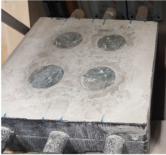
Figure 7. 21: Repaired core holes
