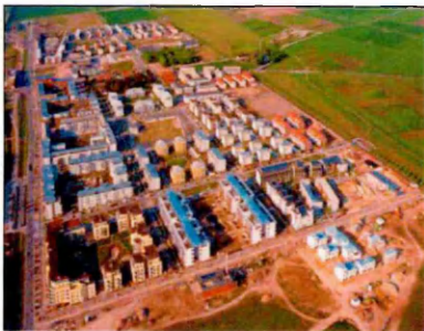
Figure 10: Residential buildings in Kronsberg (Author, 2010)
