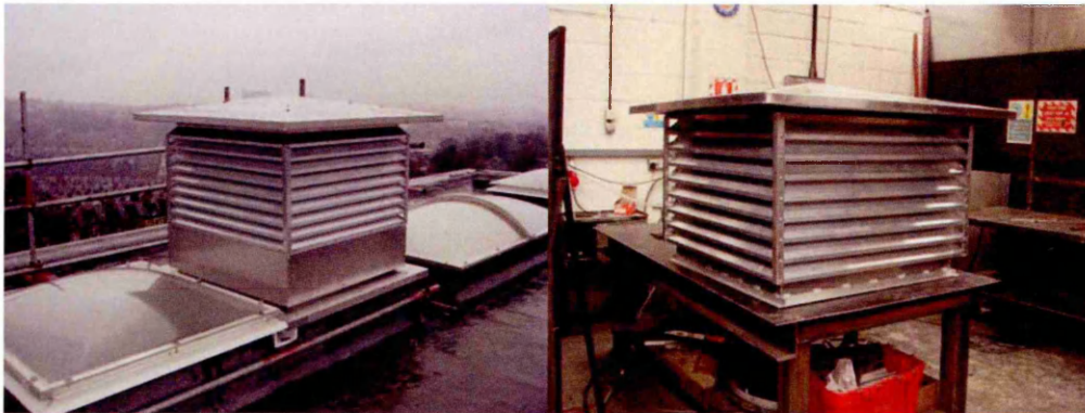
Figure 3-7 A square louvered wind vent terminal
