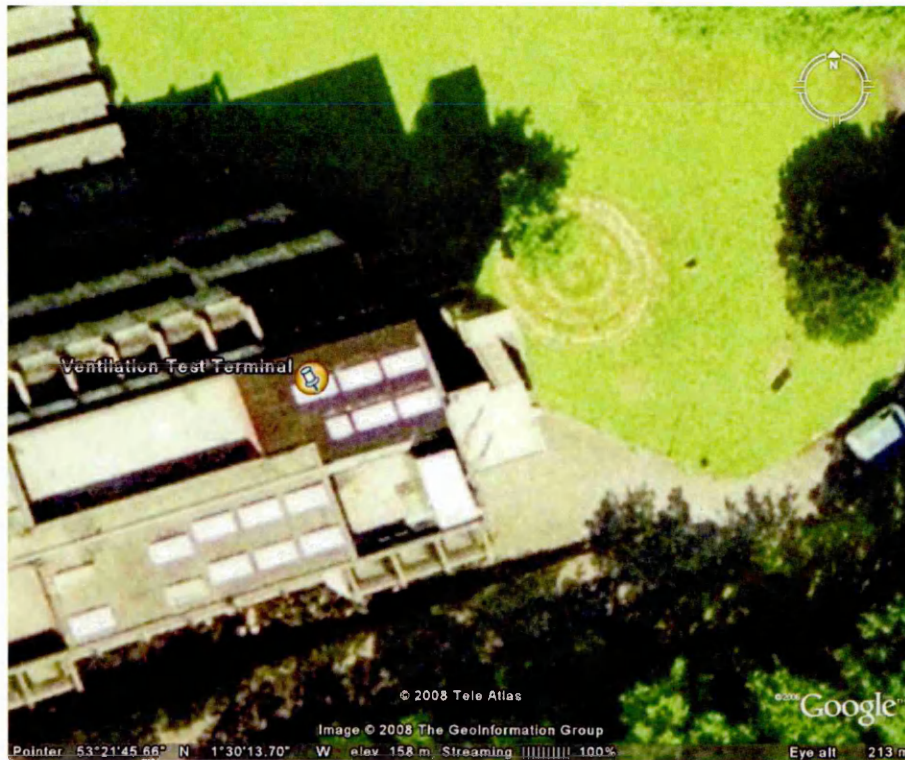
Figure 6-2 Location of wind vent test terminal on allocated building
