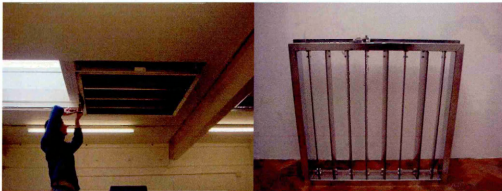
Figure 3-9 A wind vent control damper unit
