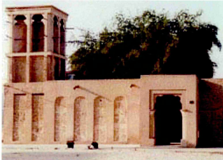
Figure 2-19 Typical wind tower in Dubai [data dubai (2007)]
