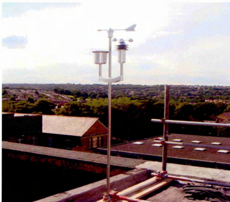
Figure 6-4 Weather station probe located on the roof
