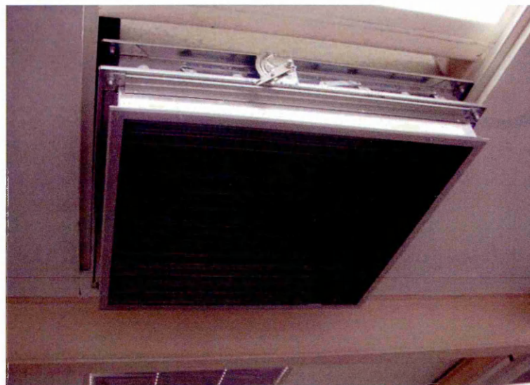
Figure 6-14 Finished internal assembly of the wind vent
