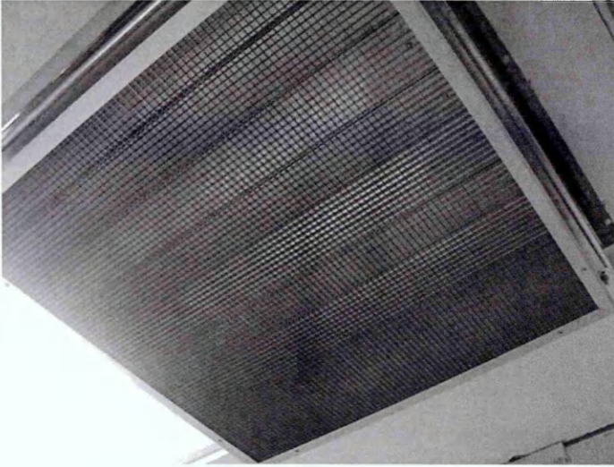
Figure 4: Shows the ventilation system with the damper in the closed position
