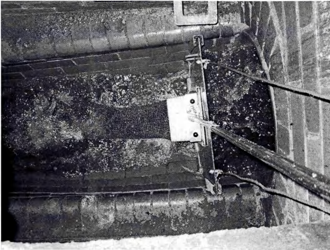
Figure 2 – Arrangement of sampling equipment with solids being collected in a mesh sack under storm conditions
