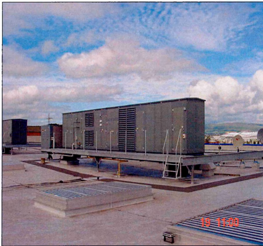
Figure 22. Large number of mechanical ventilation units
