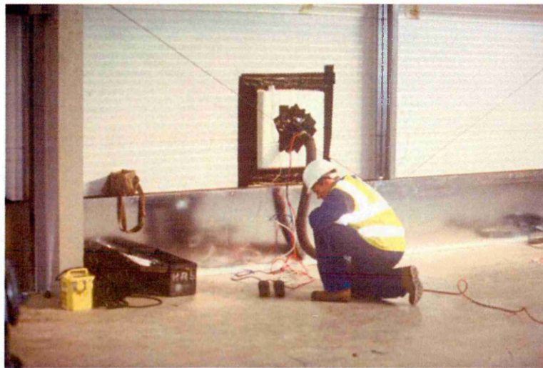
Figure 26. Joint leakage assessment by the author using a component tester
