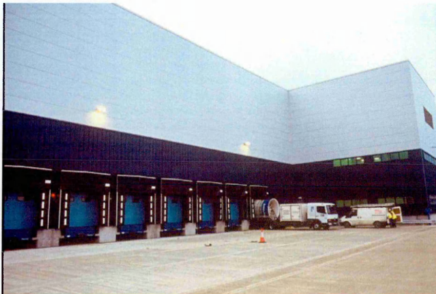
Figure 1: 2000mm diameter fan positioned in the loading bay door
