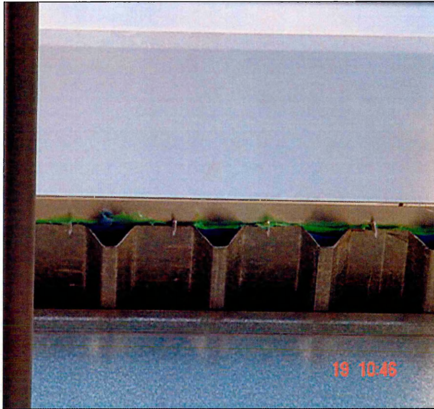
Figure 21. Lack of sealing at roof sheet detail
