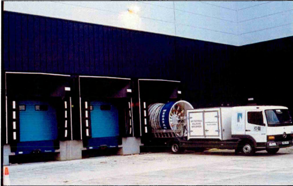
Figure 27. Megafan sealed into dock leveller entrance
