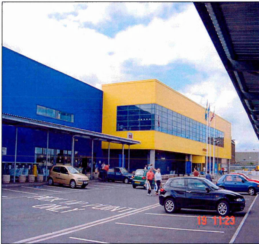
Figure 20. Building B front entrance
