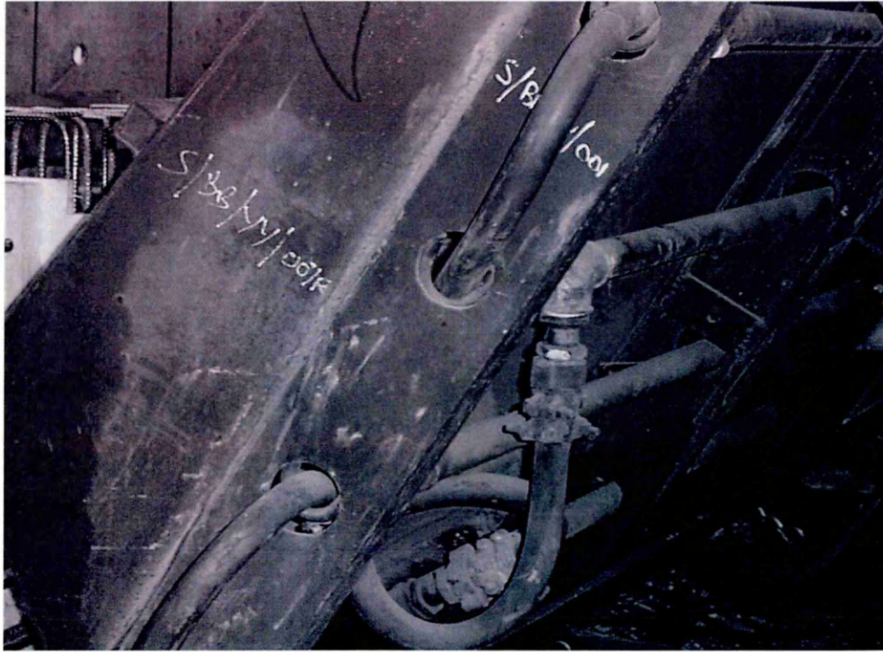
Figure 2.5. Captured steam pipe network running adjacent to steel 'Double-T' mould (picture courtesy of Tarmac Precast Concrete Ltd)
