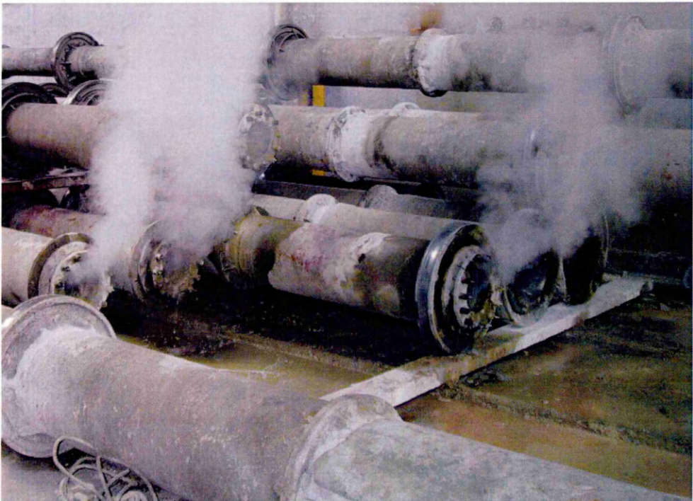
Figure 2.4. Free steam curing of prestressed pipes (Picture courtesy of Prefabet Precast Concrete Ltd)
