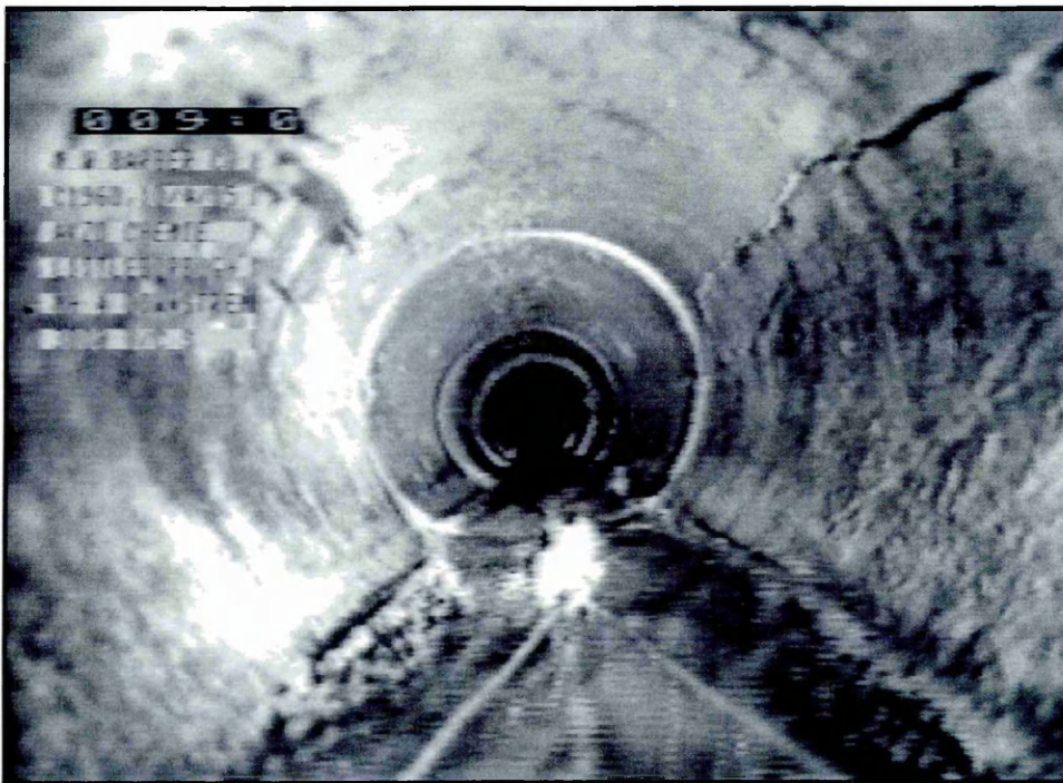
6.2(a) Crack 1 (Canny processing not applied)
