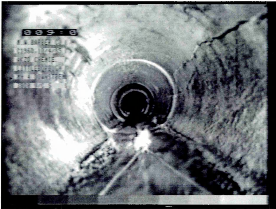
Figure 3.1 Grey-level digital image, obtained from a field CCTV survey, of a non-man-entry sewer. Three pipe junctions and a co-axial crack (top right quadrant) can be seen.
