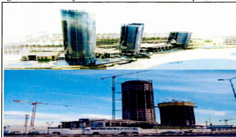
Figure 5-17: The Burj Albahar under Construction in Tripoli, 2010
