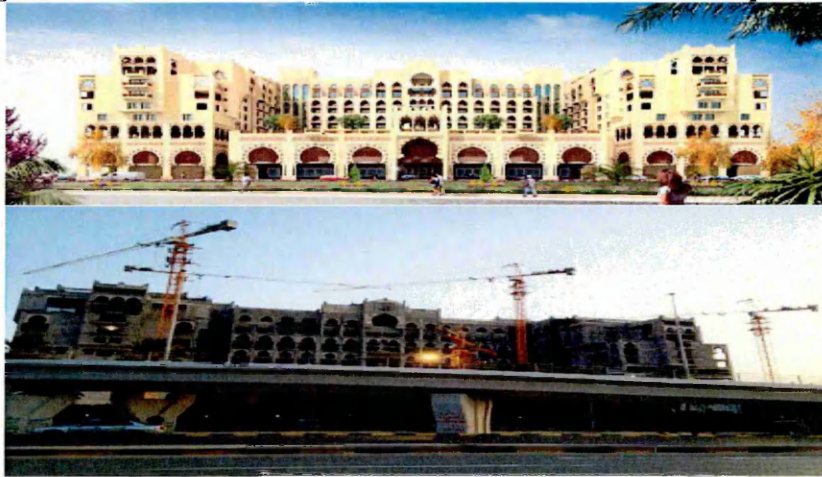
Figure 5-16: The InterContinental Hotel under Construction in Tripoli, 2010
