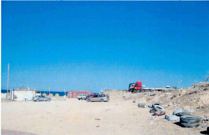
Figure 8-5: A Deteriorating Private Beach Resort in the Alkhoms City Area, 2010
