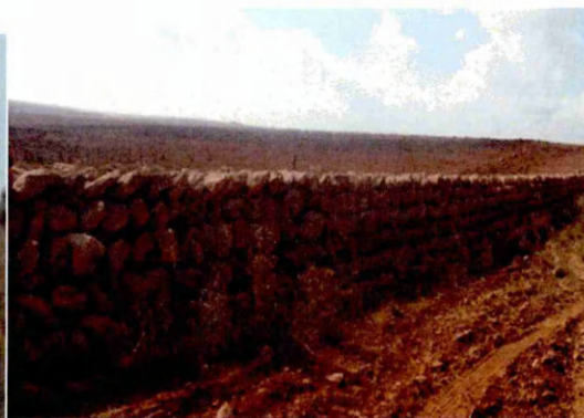
Picture 12. 2. 34. Dams about 1-1.5 m wide, 1.5 m high and 200 m long, in Marawah (09/2010). (X: 544906, Y: 3594772)
