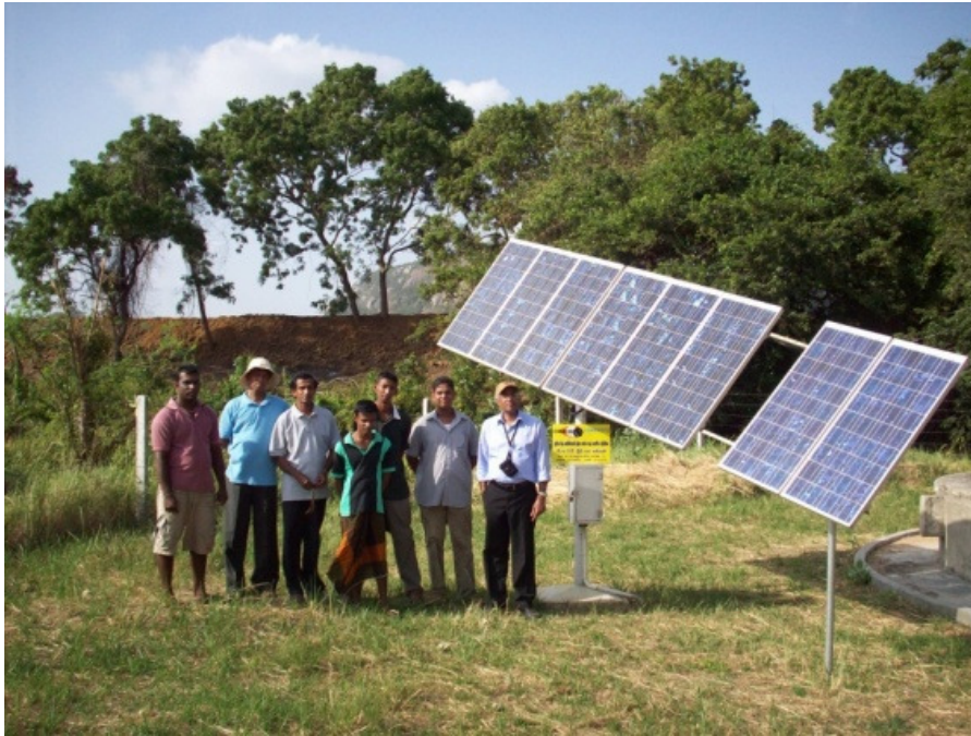
Figure 7: The pilot Solar Village started in 2008 by replacing a diesel water pump by a solar water pumping system.
