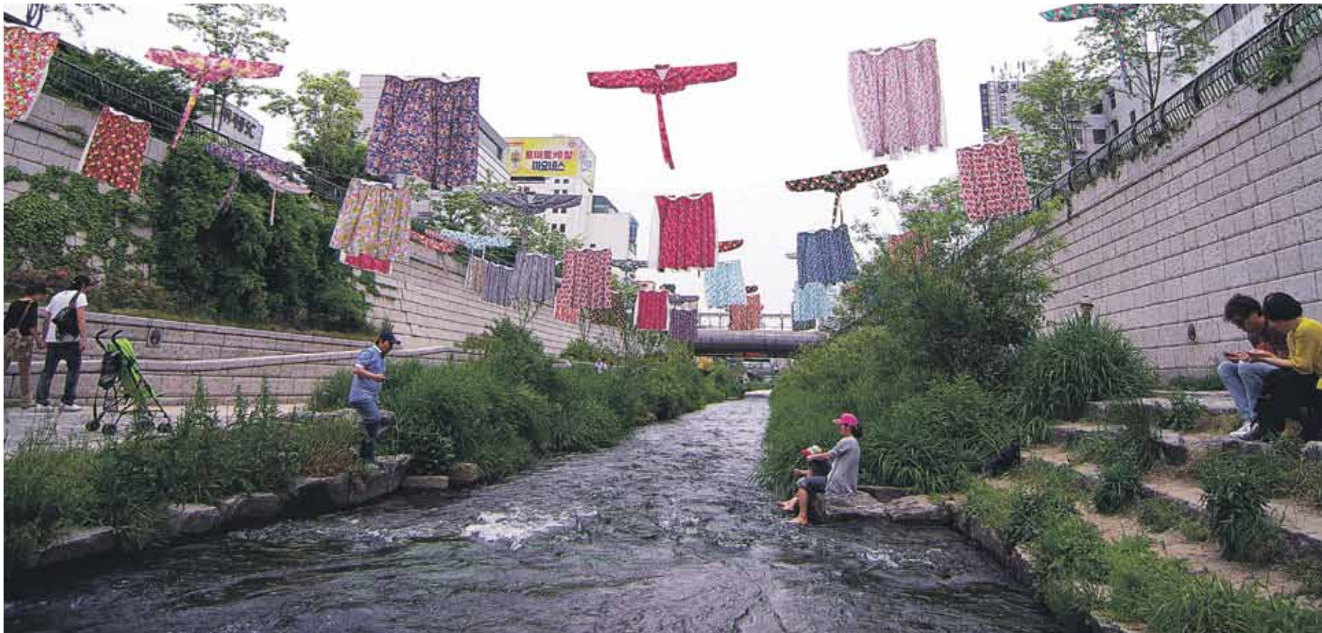
THE CHEONGGYEHEON RESTORATION PROJECT DESIGN: SEOUL METROPOLITAN GOVERNMENT (KOREA), 2005
