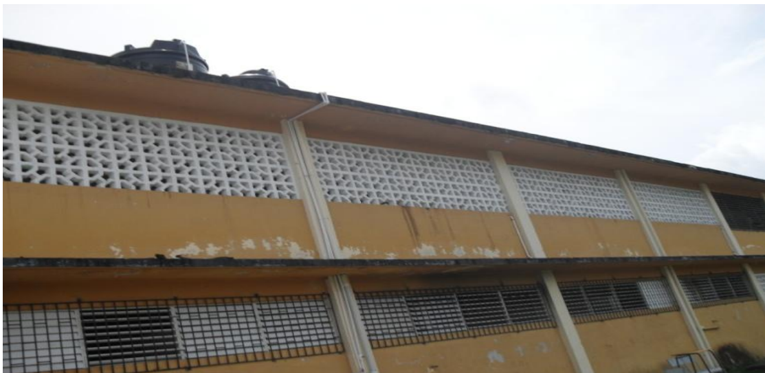
Figure 4.12. Elevation of Building with Peeling Paint.
