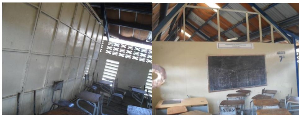
Figure 4.15. Condition of Ceiling and Ceiling with No Ceiling Bed.
