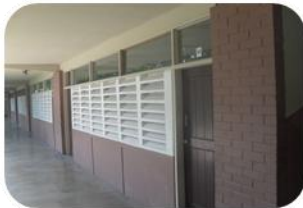
Fixed glass panels above concrete louvers
