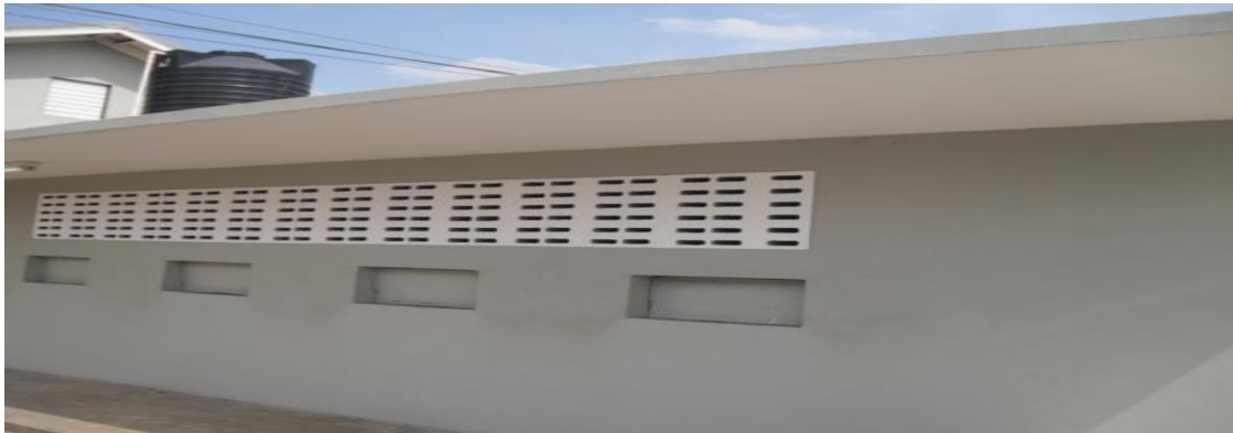
Figure 4.11. Elevation of Precast Concrete Louvers Limiting the Supply of Fresh Air and Light into Rooms.
