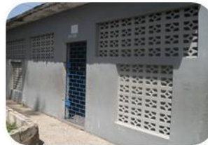
Concrete decorative blocks used as window openings. Classrooms are poorly ventilated with little admittance of light.
