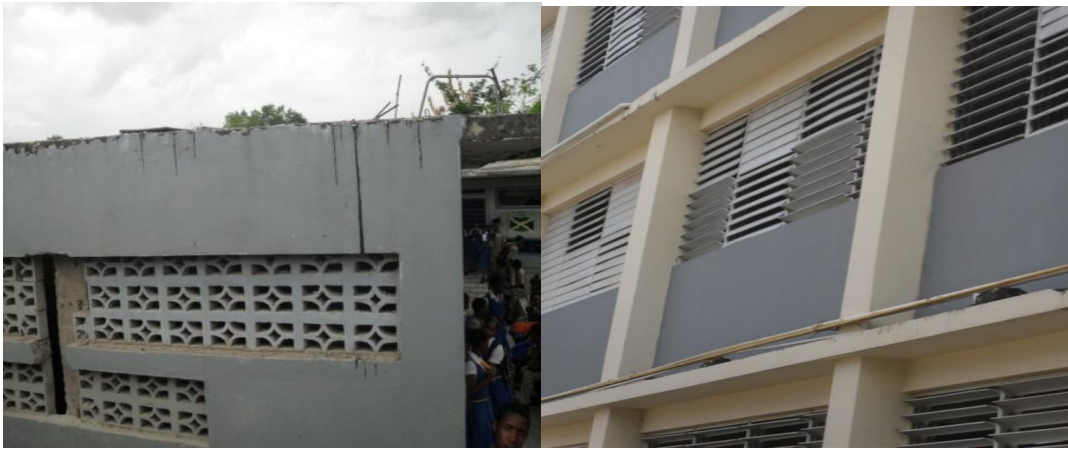
Figure 4.9. Elevation of Decorative Blocks as the Only Window Opening Contrasts with a Good Distribution of Aluminium Windows.
