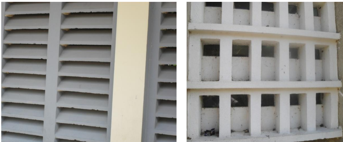
Figure 4.5. Elevation of Precast Concrete Louvers Used As Window Opening.
