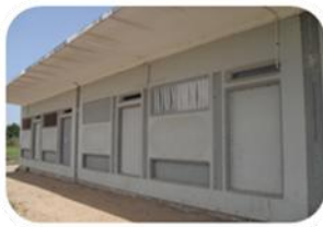
Precast structure with limited window opening. Classrooms are hot with limited light and ventilation.
