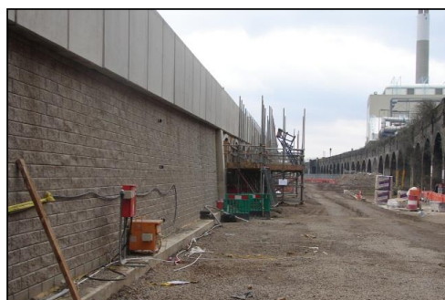
Figure 10: SS408 (Reinforced earth structure)
