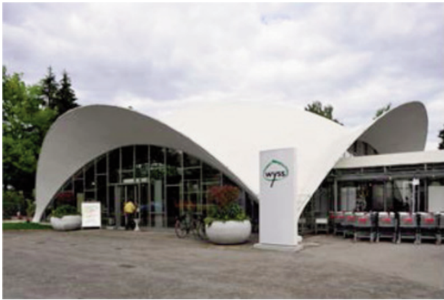
Figure 4. Wyss Garden Centre, Switzerland by Heinz Isler (1961).
