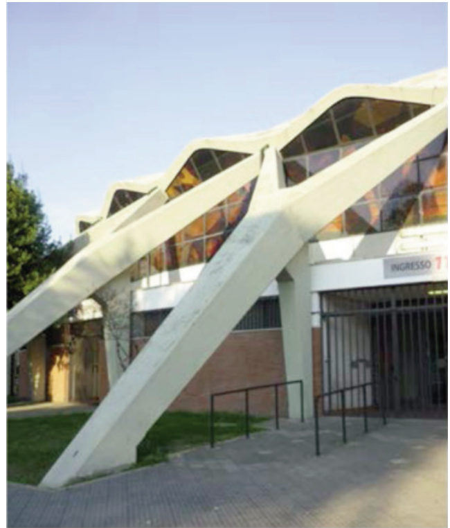
Figure 7. Y-shaped columns on the outside of Palazzettodello Sport, Rome, Italy by PL Nervi (1956–1957).
