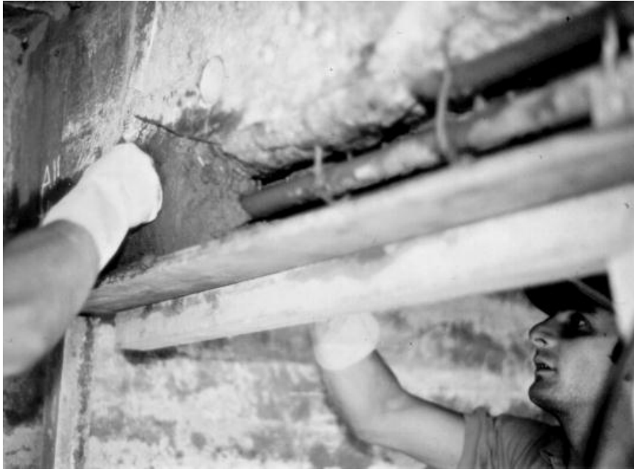
Figure 3: Hand applied repairs to beams at Gunthorpe Bridge (unpropped structure)
