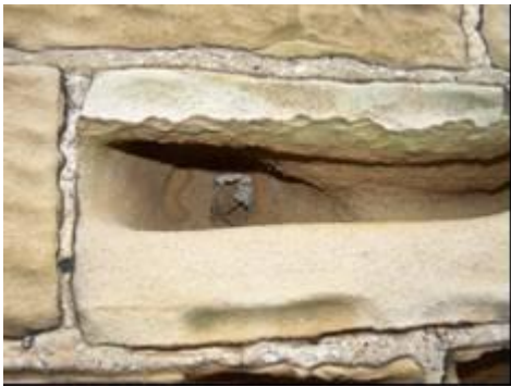
Figure 3: Example of cavernous weathering, southern elevation Norwood Piggeries
