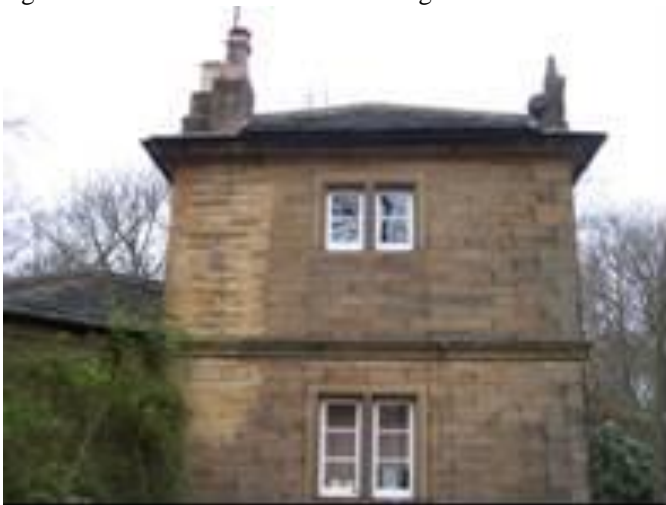
Figure 5: Stone decay along route of flue
