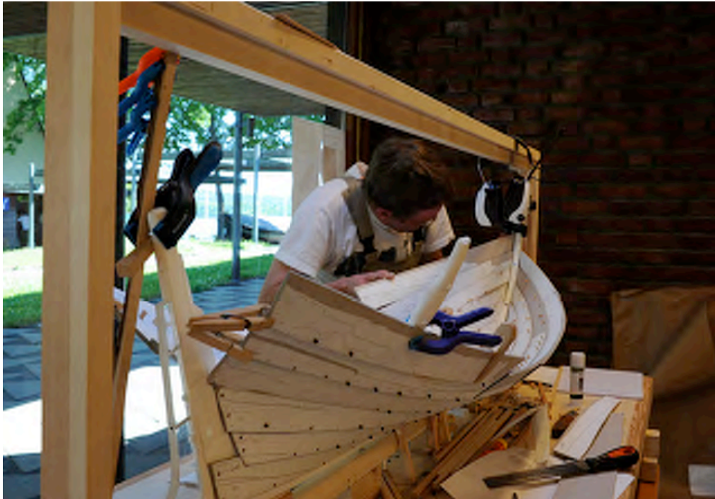
Fig 2: The boat builder in the process of making a 1:5 model in cardboard based on the excavated fragments. This model becomes then a basis for building a full scale replica.
