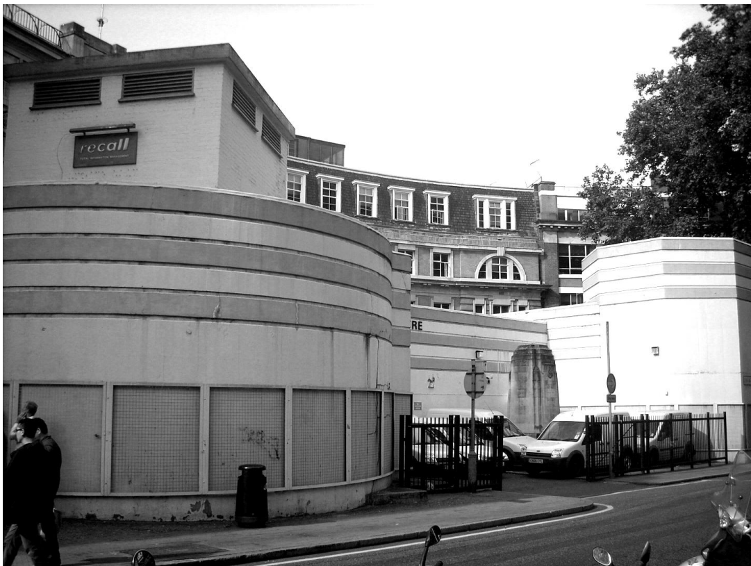
Eisenhower's 'deep shelter', Goodge Street, London – now Channel 4's archive.
