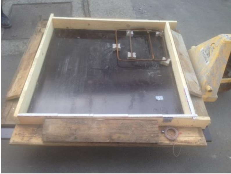
Figure 9.12: Placement of steel reinforcement links prior to casting.
