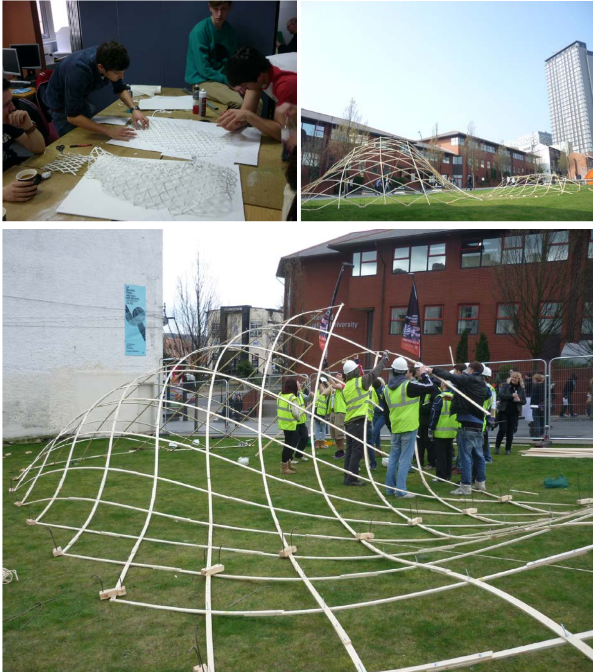
Figure 3: Physical models of timber gridshells were made from paper card strips (top left). The Swell timber gridshell (top right) on display for 2 weeks in Sheffield City Centre in 2011. Students create the shells together to learn and understand timber as a material in bending and deformational behavior arising from forces applied. (Bottom) [credit: Gabriel Tang]
