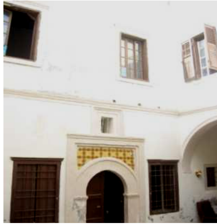
openings towards a courtyard
