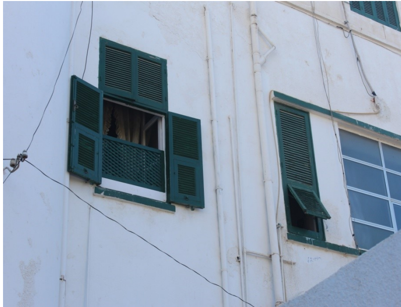
Figure 6.13: Ka-Zalanges/Type-A: The use of wooden-lattice/ mashrabiyya for sight privacy Source: Author field-work
