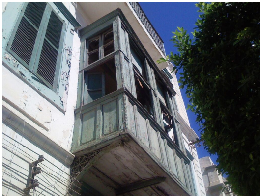
External screened window ( Mashrabyyah ).
