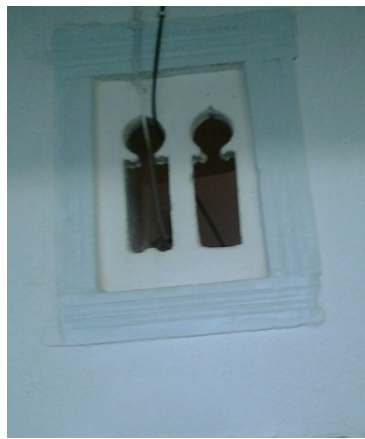
Details: internal screened window
