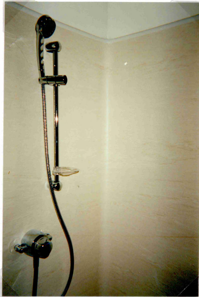
Figure 6.6: Corner of shower area.
