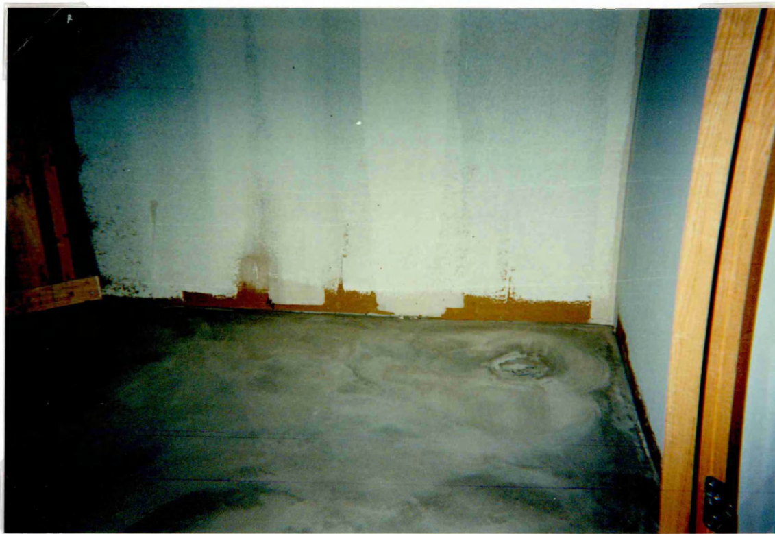
Figure 6.7: Floor screed to shower area
