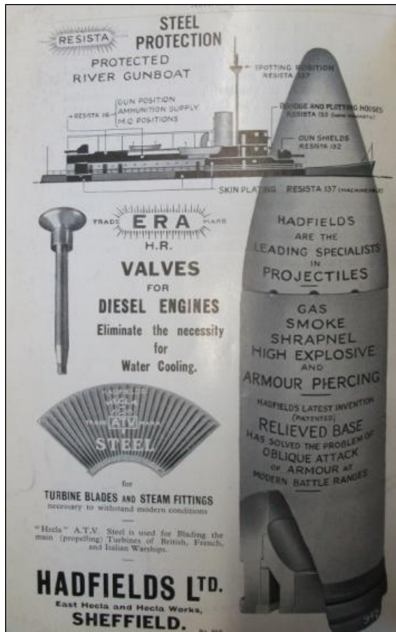
Figure 5.2: Hadfields' Advert from 1934, showing the relief base design. Taken from 'Note on the New Armour Piercing Projectile', reprinted from Brassey's Naval and Shipping Annual 1934.
