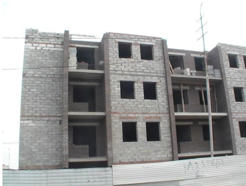
Figure 6.3: Hidden issues, inappropriate methods of buildings' construction in the harsh climatic conditions of Yamal
