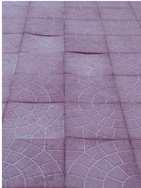
Figure 6.2 (a): Hidden issues, inappropriate construction of the pathways in Yar-Sale, Yamal, YNAO
