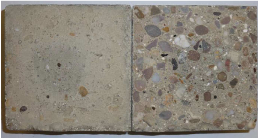
Fig. 3 Typical failure at the bonded interface between substrate and repair material
